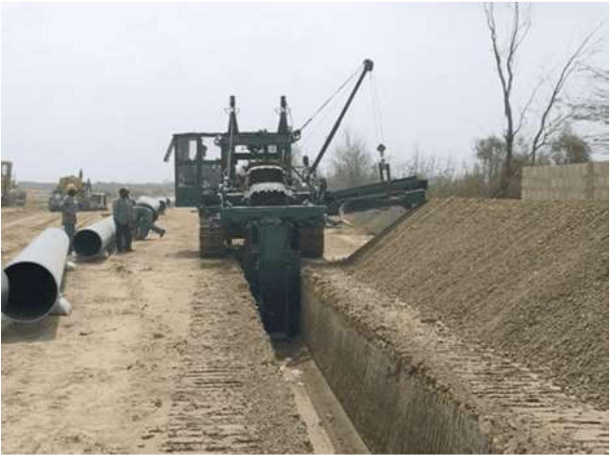
Figure 9 - Pipe trenching machine
