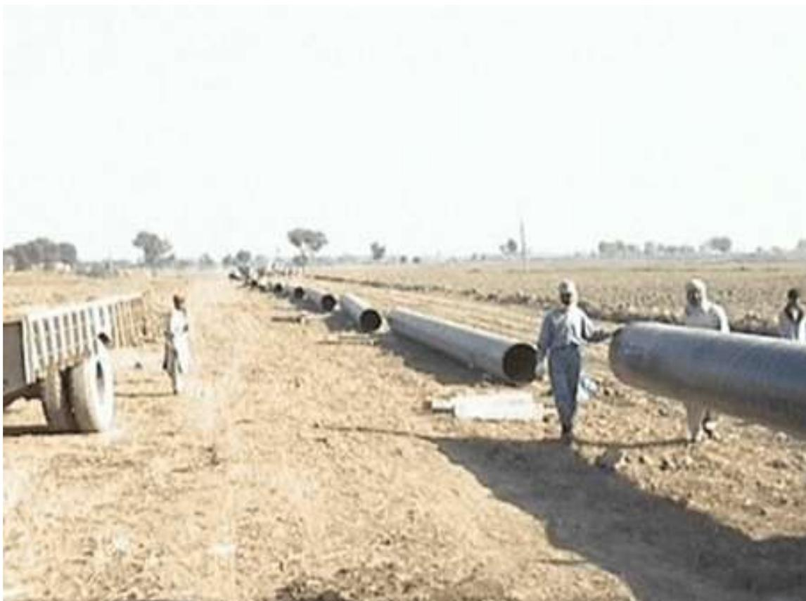
Figure 12 - Stringing of 26-inch diameter pipe
