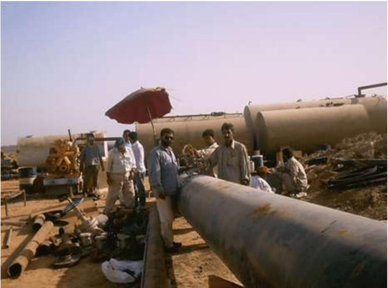
Figure 23 - Water tanks for hydrostatic testing
