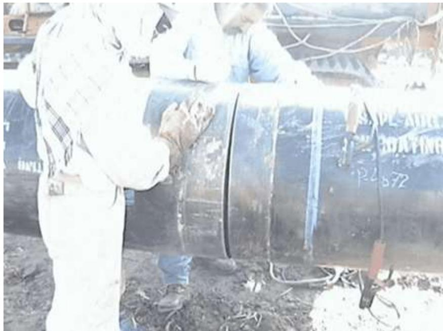
Figure 13 - Preparation for welding
