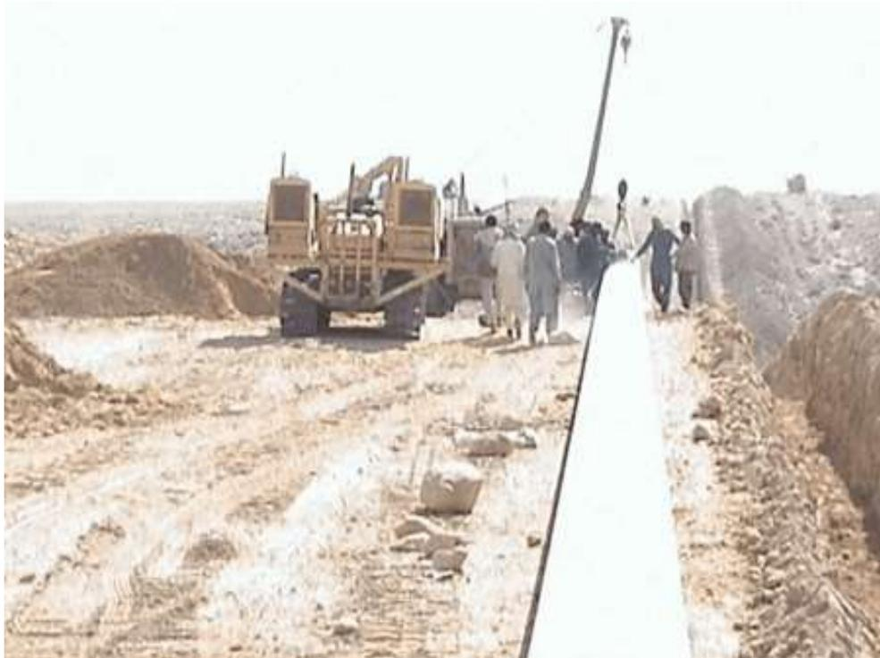
Figure 19 - Welded section lowering at the construction site
