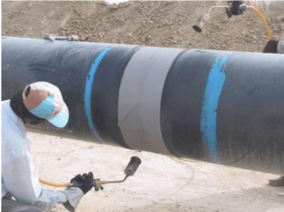
Figure 17 - Flame of burned natural gas on sleeves
