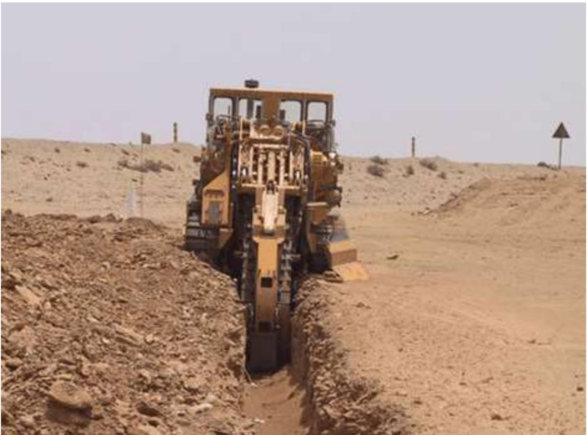
Figure 6 - Pipeline trench in rocky soil area
