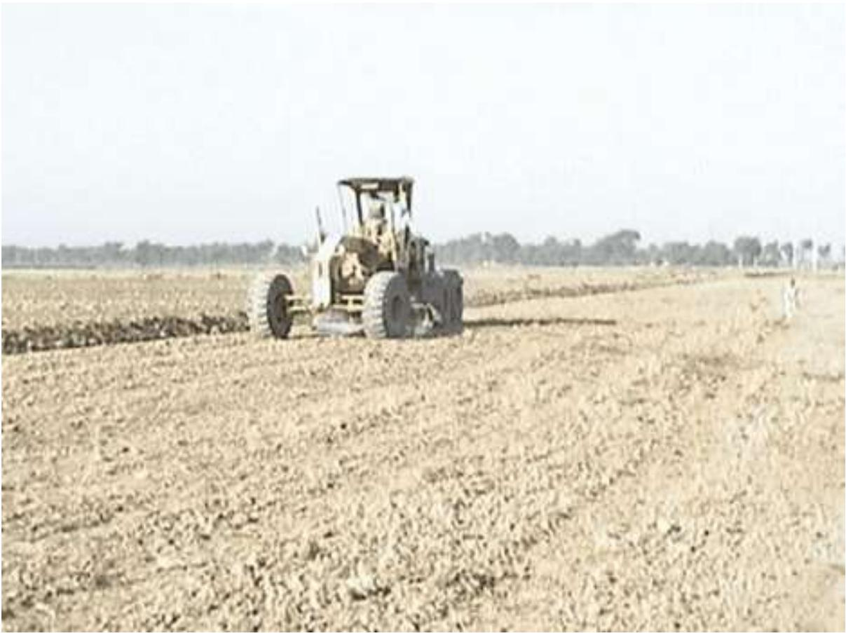
Figure 3 - Grader is clearing the right-of-way (ROW)
