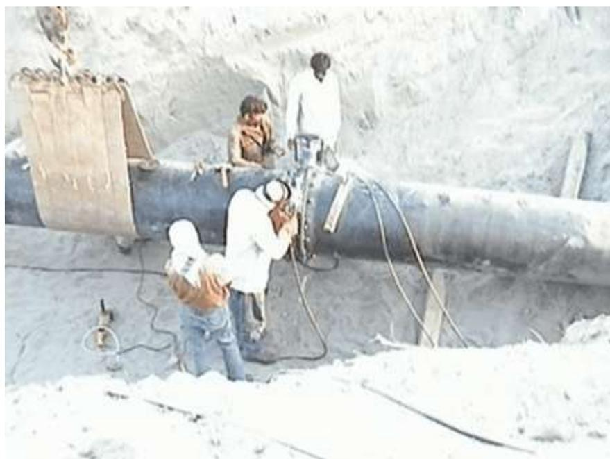
Figure 14 - Shielded metal arc welding of line pipe
