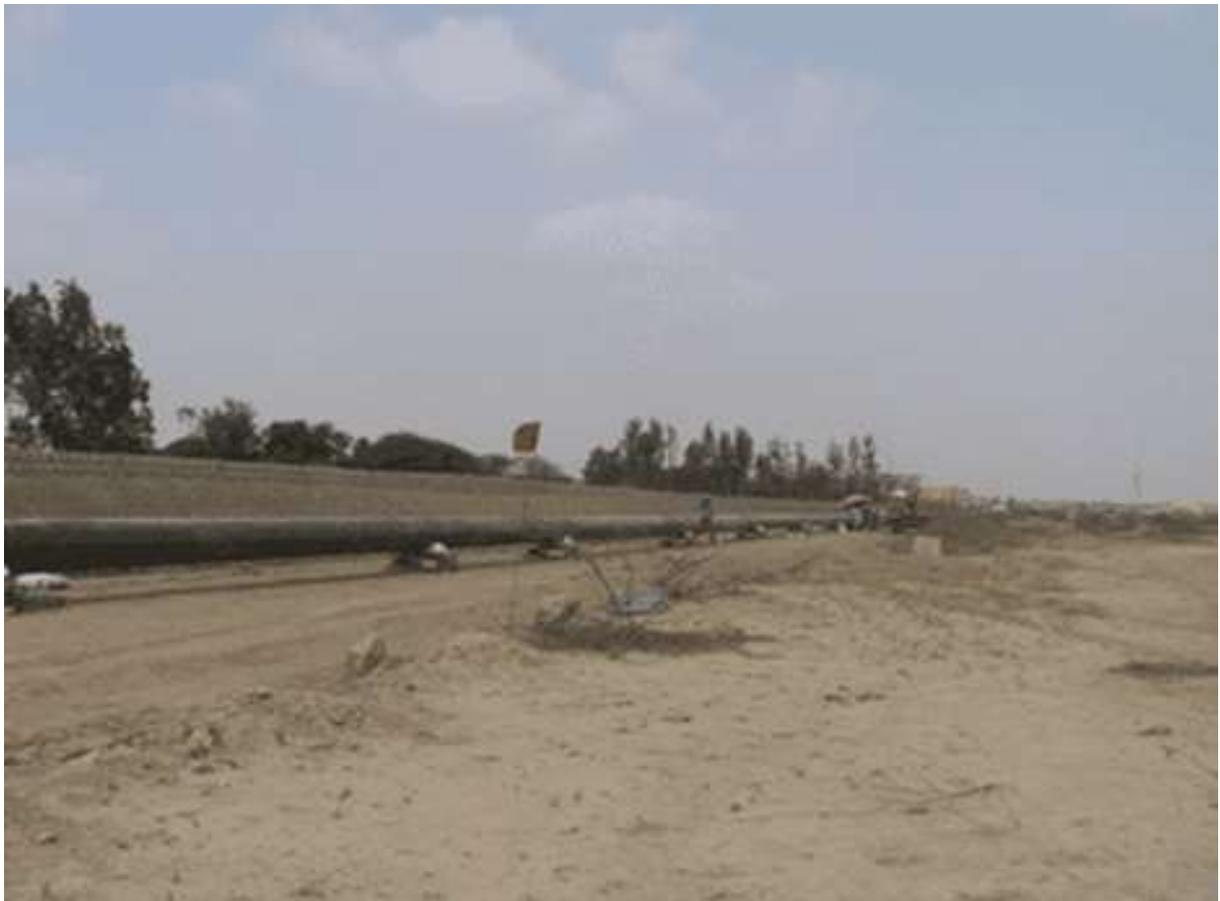
Figure 16 - Continuous welded section of line pipe
