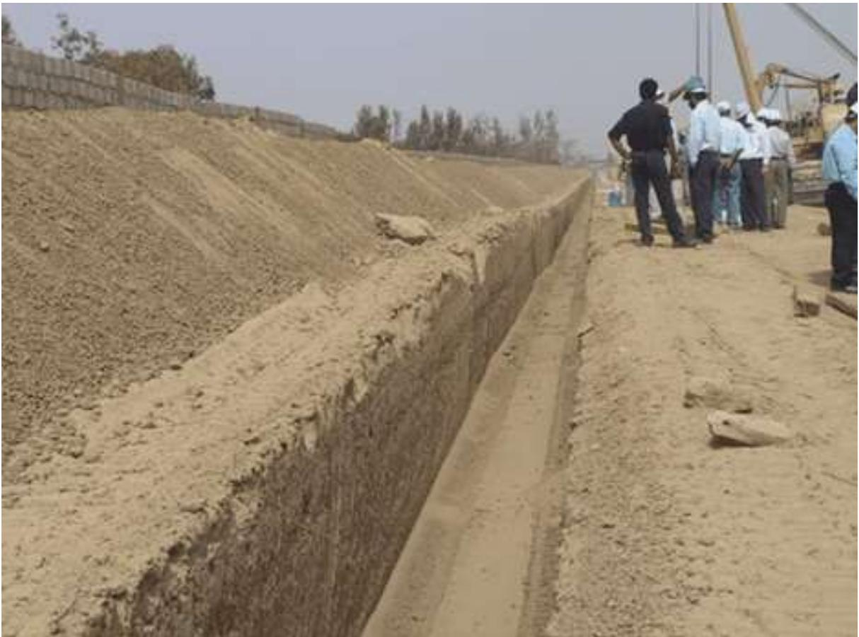
Figure 10 - Pipe trench in soft soil
