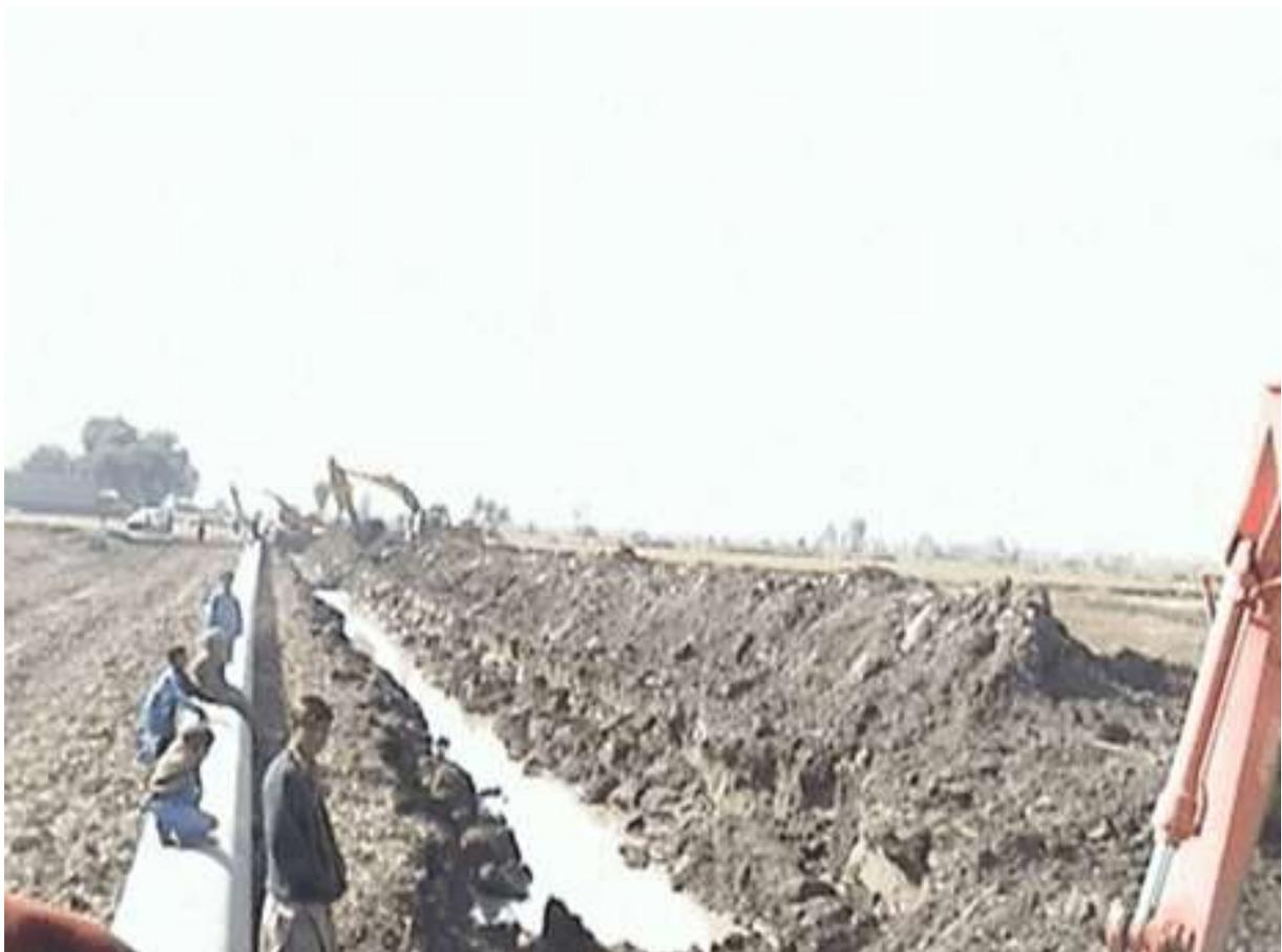
Figure 8 - Water-filled pipe trench
