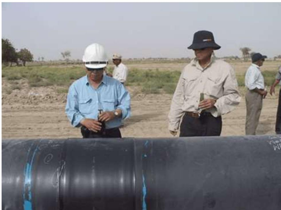
Figure 18 - Heat Shrink Sleeve on joint
